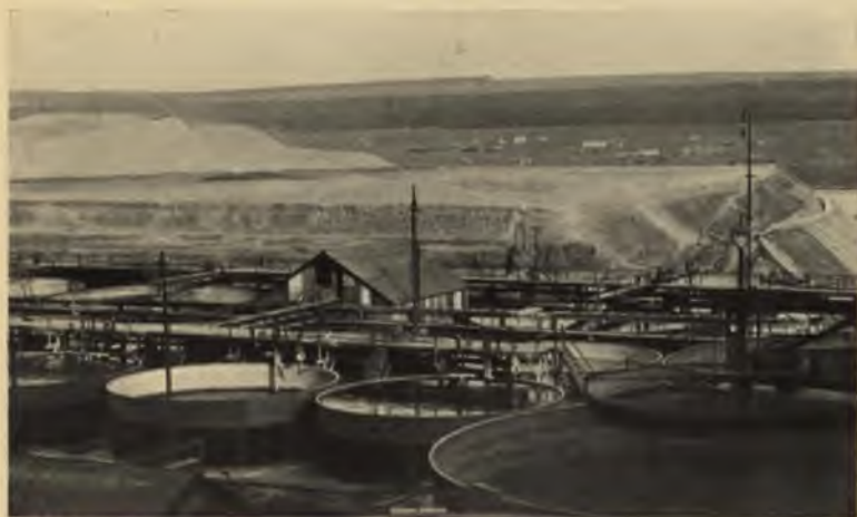
VIEW OF CYANIDE WORKS
